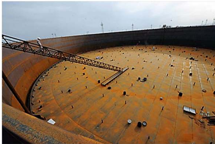
Figure 4. One of the biggest storage FR tank with a capacity 100,000 cubic meters (Northwestern China's Xinjiang Uygur Autonomous Region).
