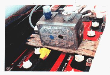
Figure 19. General Monitors hydrogen concentration sensor positioned above batteries in the FireFly<sup>™</sup> 600 battery enclosure.
