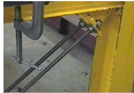
FIGURE 2: CLOSE-UP OF BEAM-COLUMN CONNECTIONS.
