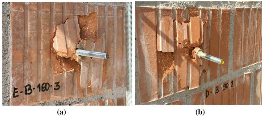
Fig. 7 Combined sliding failure and block cone failure (a) and combined sliding failure and block failure (b)
