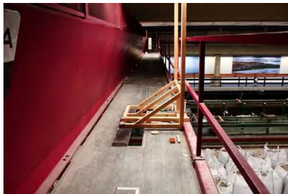
Figure A.3: The camera was installed on a frame on the crane.
