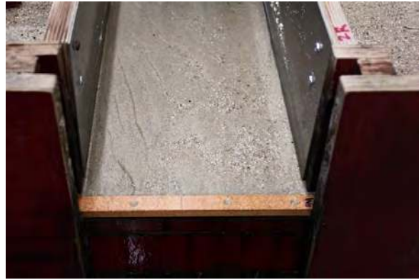
(b) Downstream installed weir
