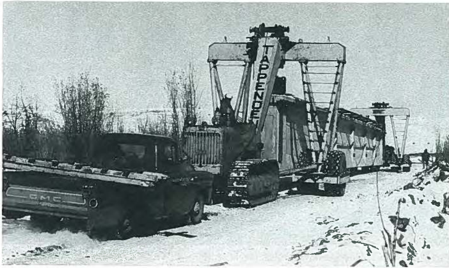
Fig. 27. Handling the 148-ft (45.1 m) post-tensioned girders for the Duchess Bridge on Highway 36 across the Red Deer River.
