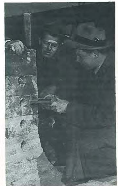
Fig. 49. The author (right) and his brother Thomas Anderson checking concrete strength of abutment with Schmidt test hammer (1951).
