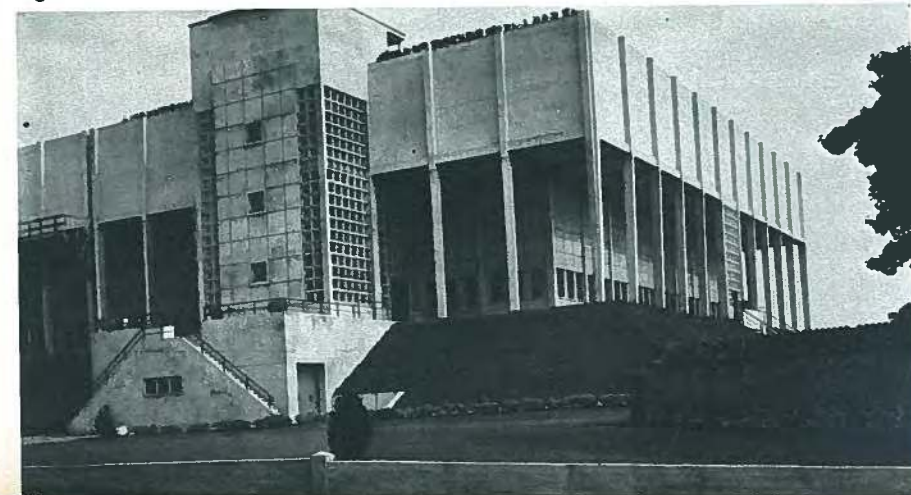
Fig. 31. Water storage reservoir and offices, Orleans, France.
