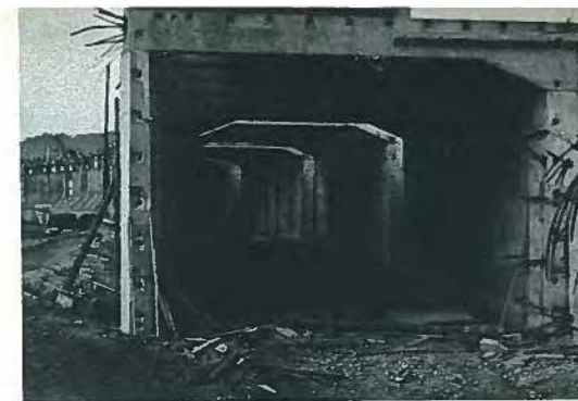
Fig. 30. Covered viaduct under construction, Rouen, France.
