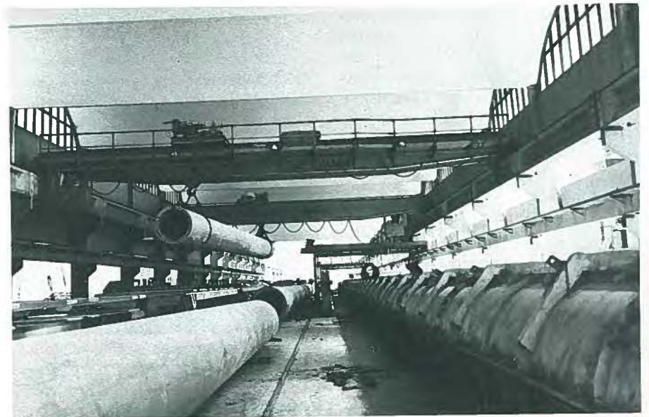
Fig. 84. Freshly cast prestressed hollow cylinder piles.
