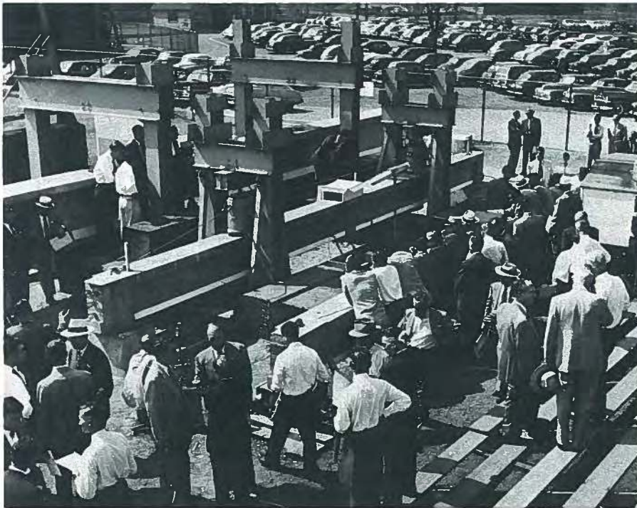
Fig. 37. An overflow crowd of invited guests witnessed the Austin Company tests in 1951. Three full-scale girders [two 40-ft (12.2 m) and one 60-ft (18.3) girders] were load tested using hydraulic jacks.
