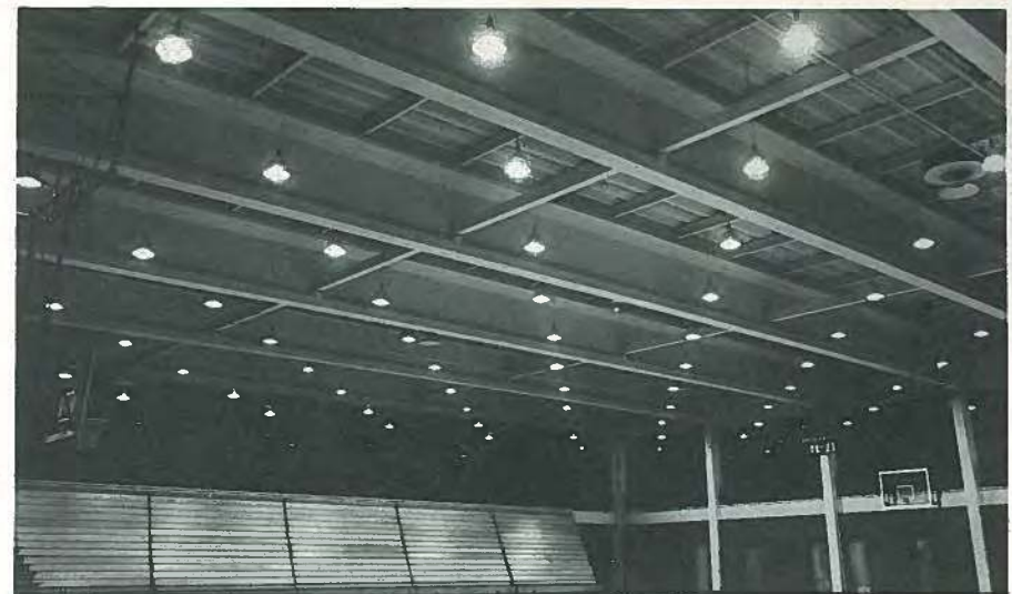
Fig. 42. Completed gymnasium with 120-ft clear span.
