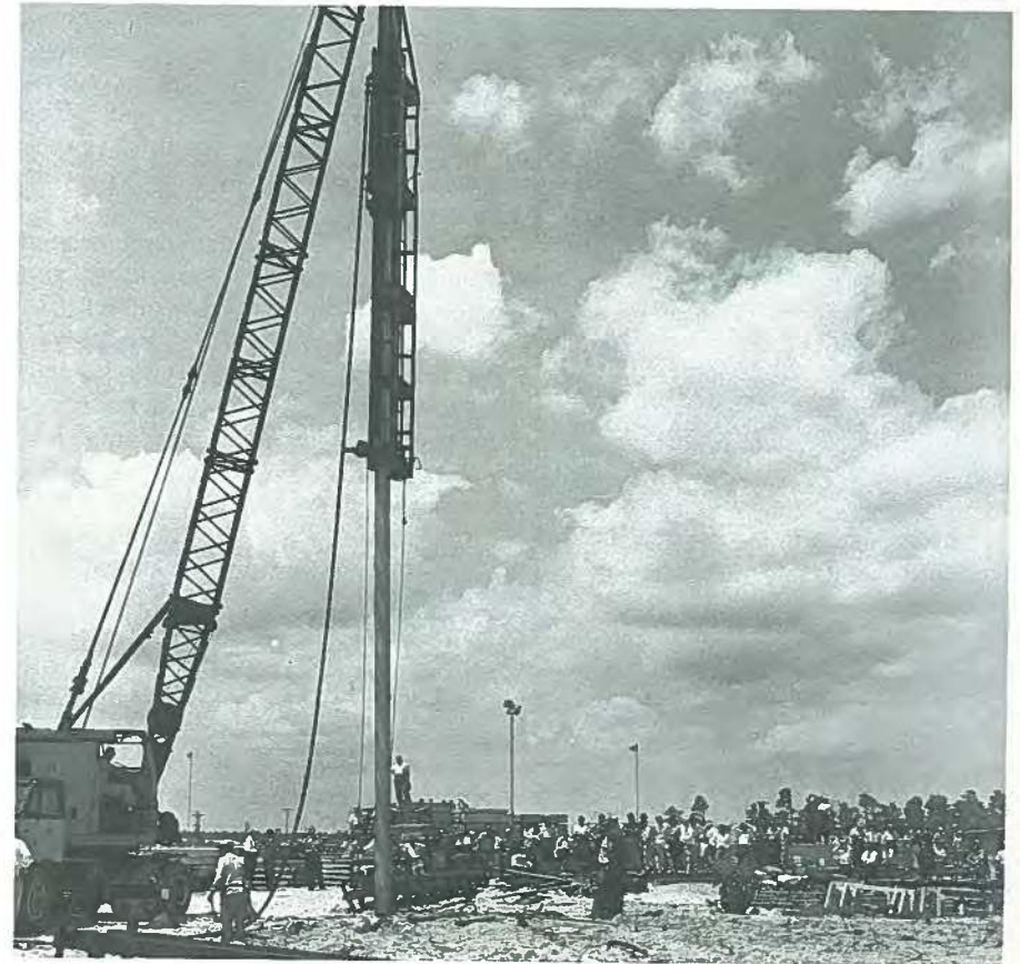
Fig. 31. Pile driving demonstration test at Cone Brothers Construction Co.
