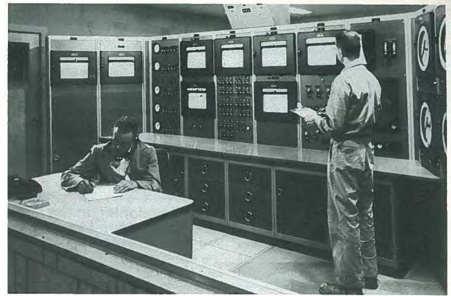
Fig. 38. Operating console in PCA's fire test center.
