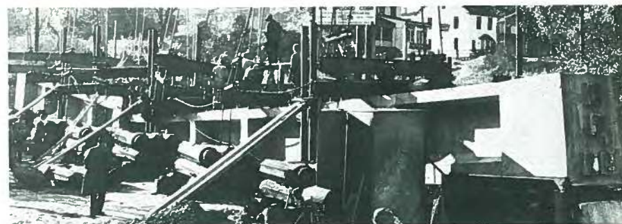
(c) Girder after failure.
