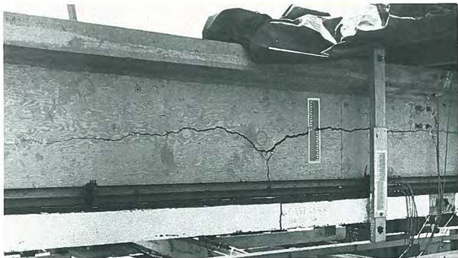
Fig. 39. Crack pattern in 40-ft (12.2 m) prestressed girder (P-40) using external unbonded tendons. The crack originated at midspan at bottom flange running up to the centroid of the girder and then branching out horizontally because no web steel was provided (Austin Company tests).
