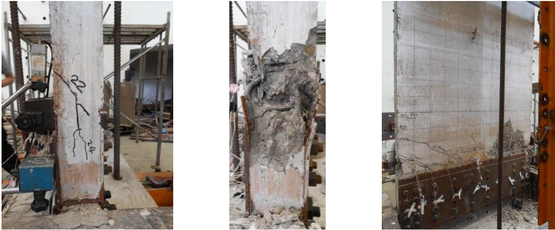
(a) Vertical cracks at compression end (b) Compressive failure (c) Overall failure mode
