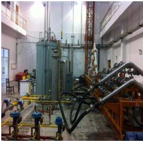
Figure 1. The multiphase pipe flow laboratory
