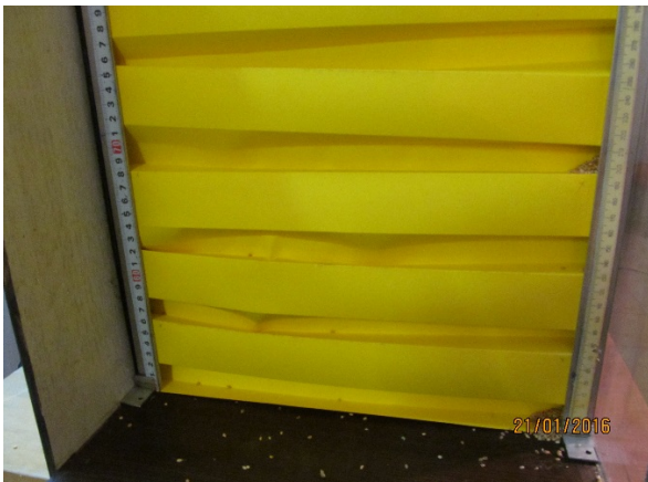
Fig. 6. Panel destruction due to loss of local stability of bottom plates of the second and the third corrugations
