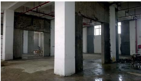
FIGURE 10: View of short-pier shear walls.
