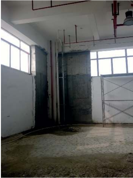
FIGURE 1: Photo of a short-pier shear wall.
