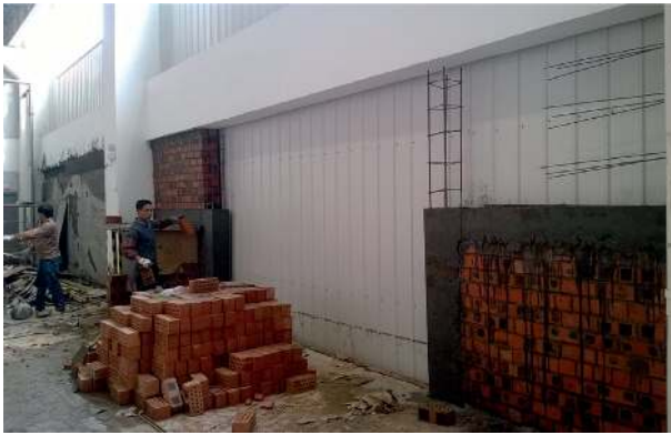
FIGURE 9: Short-pier shear walls in construction.
