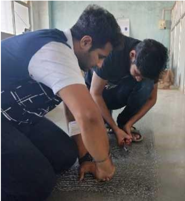
Fig. 3: Ferrocement- Application of Cement Mortar IV.
