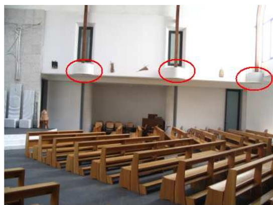
Fig.7: Side speakers position and geometry in the church under study
