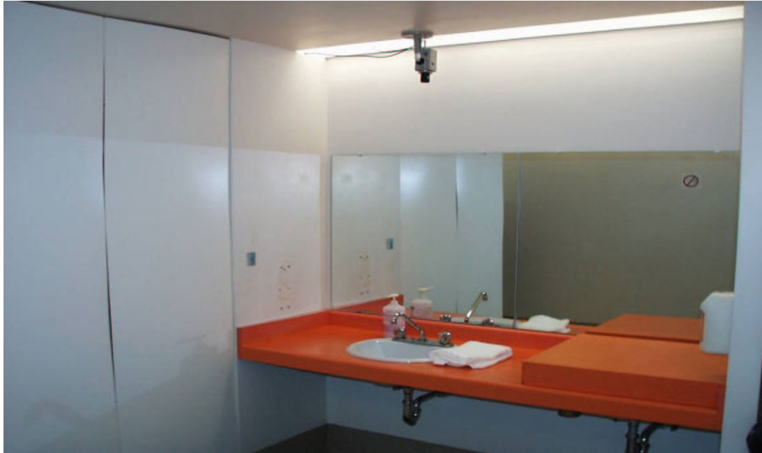
Figure 5.4: Retrofitted bathroom at the Sunnybrook hospital in Toronto for the COACH project.
