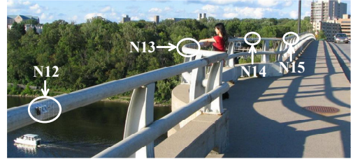
(b) On-site View
