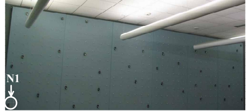
(b) On-site View
