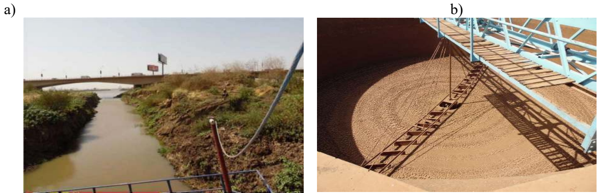
Fig. 8 Impacts of sedimentation problem: a) Narrowed river width near Shambat Bridge on the Main Nile due to accumulation of sediment and b) High turbidity level during the water treatment process at Bait Elmal Water Treatment Plant (Photo: Gore, March 2015).
