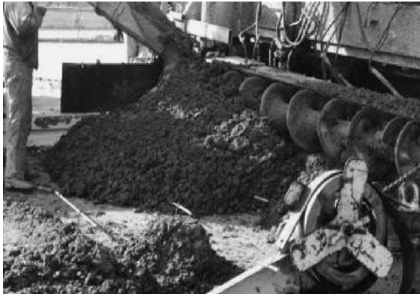
Figure 2.9 Use of Slip Forms (Rasmussen and Rozycki 2004)
