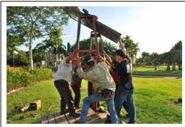
The frame being attached to the column
