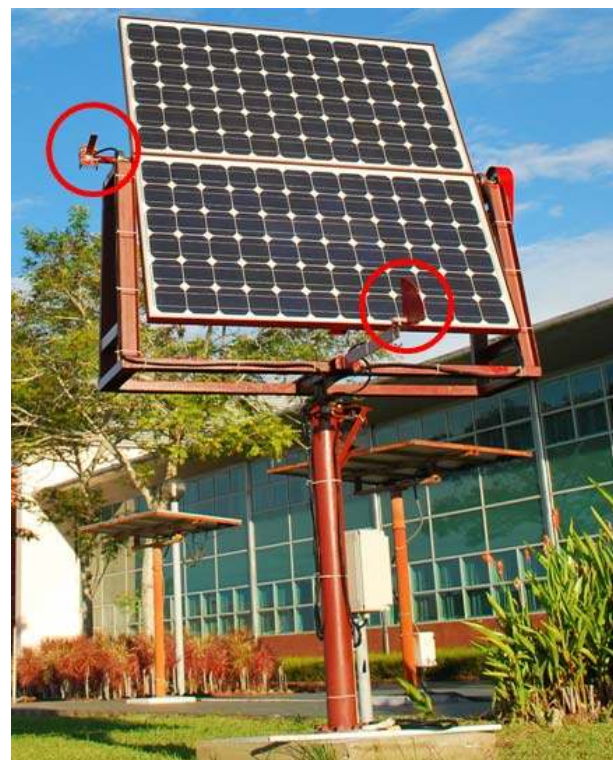
Figure 14. Placement of the sensors on the structure.
