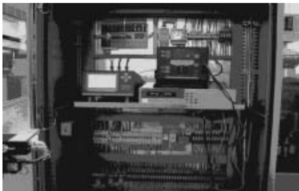
Fig. 1 The Transformer Diagnostic System
