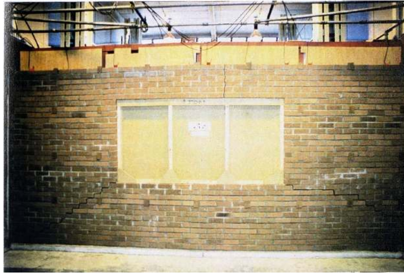
Figure 10: Crack patterns in the experimental study (SB02)
