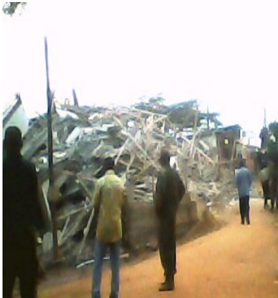
Figure 1. Building collapse at Elig-essono Suburb, Yaoundé
