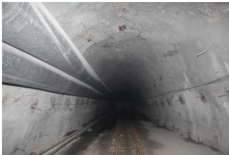
FIGURE 17: The roadway with new supporting design.
