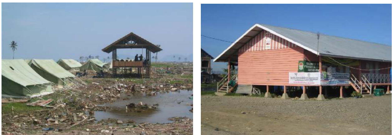
Figure 6: Emergency shelters (canvas tents) versus transition accommodation (wooden barracks). The canvas began to degrade in the tropical conditions very quickly, making the transitional versus permanent debate rather urgent (Images from Steinberg 2007, 154).
