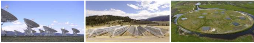
Fig. 9 Examples of radio interferometers used to search for FRBs (from left to right): the Jansky Very Large Array (JVLA) of 2725 m dishes in New Mexico, USA, the Canadian Hydrogen Intensity Mapping Experiment (CHIME) with four cylindrical paraboloids each 100 m long and 20 m in diameter in British Columbia, Canada, and the core of the Low-Frequency Array (LOFAR) of dipoles in the Netherlands
