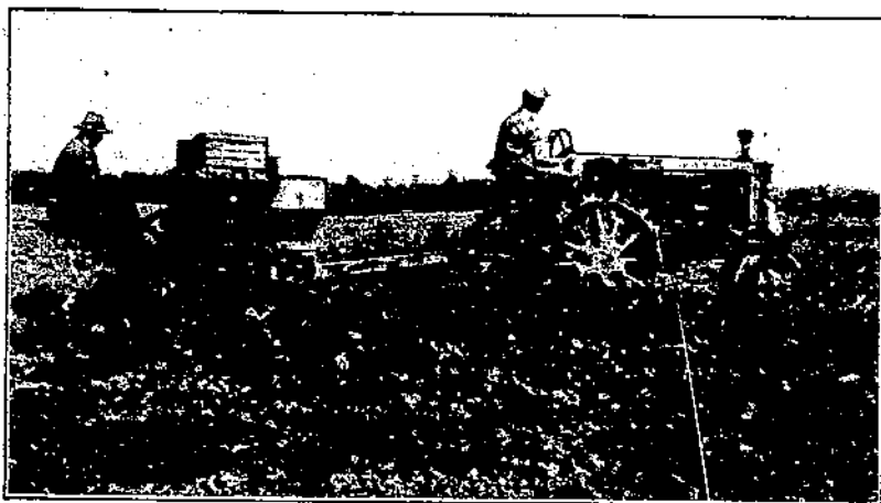
FIGURE 3.—Combined potato-planting and fertilizer-distributing machine of the two-row tractor-drawn type.
