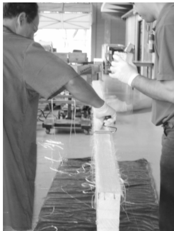
Application of fiberglass fabric.
