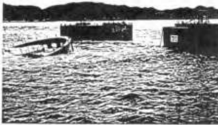
Photo. 1 Slid Caisson in Sakai Port
