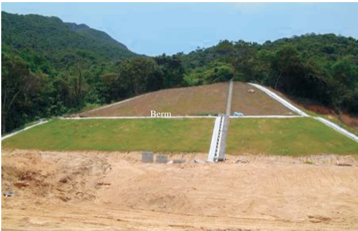
Fig. 4. Site photograph showing the cut slope and hillside slope condition after road excavation in December 2001.
