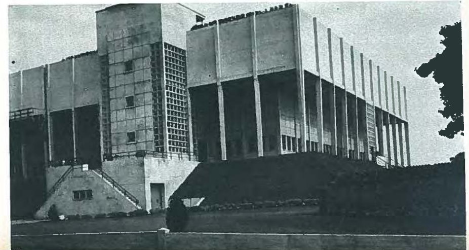
Fig. 31. Water storage reservoir and offices, Orleans, France.
