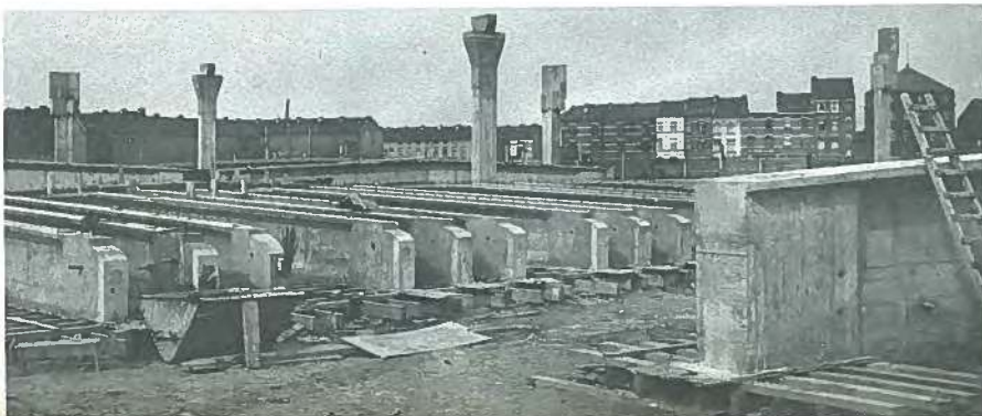
Fig. 33. Construction site of prestressed warehouse in Ghent, Belgium. The beams, cast on location, are ready to be hoisted into position.
