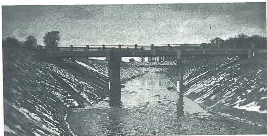
Fig. 10b. Completed three-span block-beam bridge in Tennessee.
