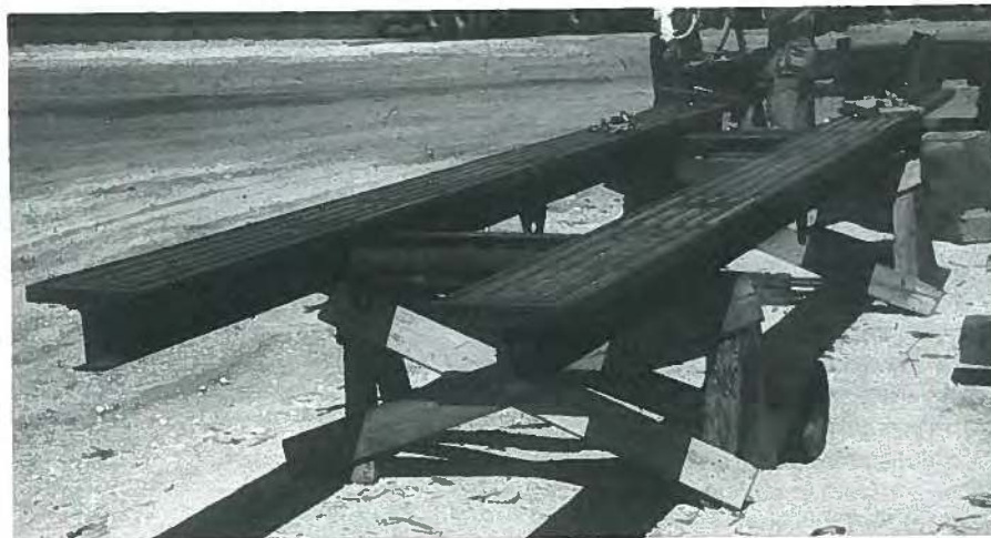
Fig. 24. Vacuum lifter used in 1953 for Loyola University's stadium seats in the upside down position. Note that the sponge rubber strips will be compressed by atmospheric pressure when a vacuum is applied between the lifter and the top of the slab. Thereby, the lifter pushes against the concrete panel sufficiently to allow it to be removed from the mold, just as a giant suction cup would.
