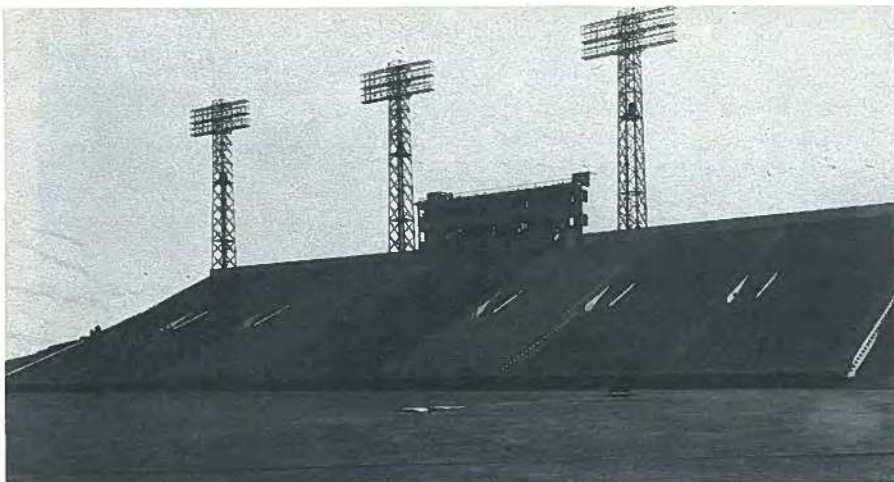
Fig. 25. The original 20,000 seat McMahon Football Stadium in Calgary, completed in 6 weeks in 1960.
