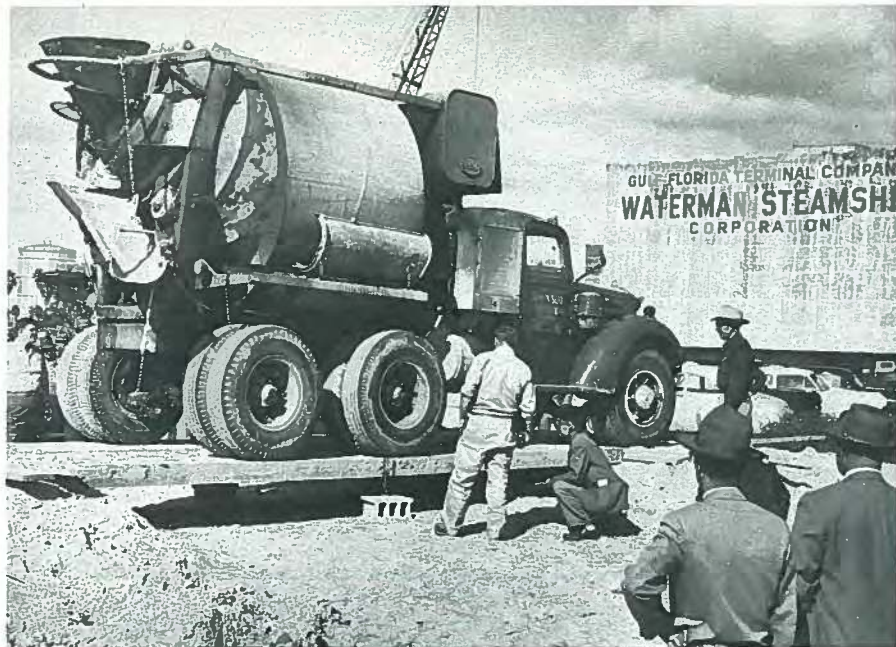
Fig. 24. Demonstration test by Cone Brothers Construction Co. in Tampa, Florida (1954) of 2-in. (51 mm) thick prestressed slab with 4-in. (102 mm) composite topping. The span was 30 ft (9.2 m) long.
