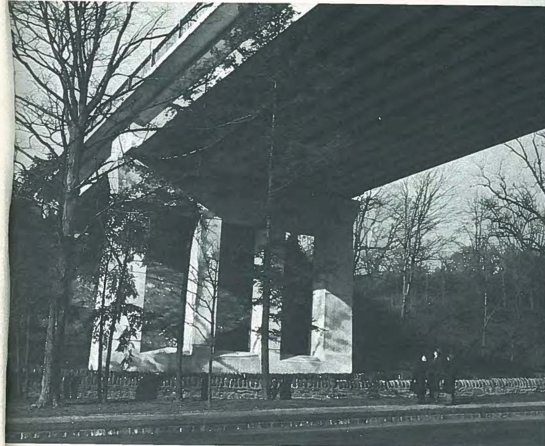
Fig. 20. The completed Walnut Lane Bridge and the men responsible for its construction; (from left to right) Prof. Magnel, Samuel Baxter (ASCE) and Charles Zollman (author of this paper).
