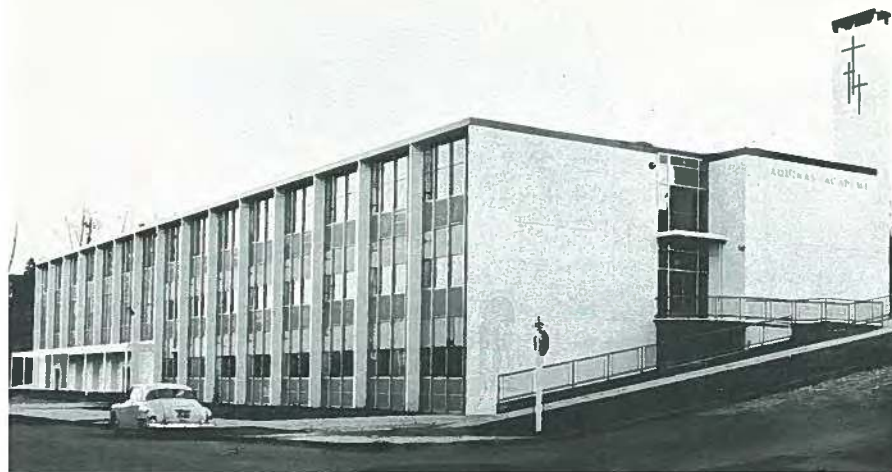
Fig. 67. Completed school, after only 6 months of construction.
