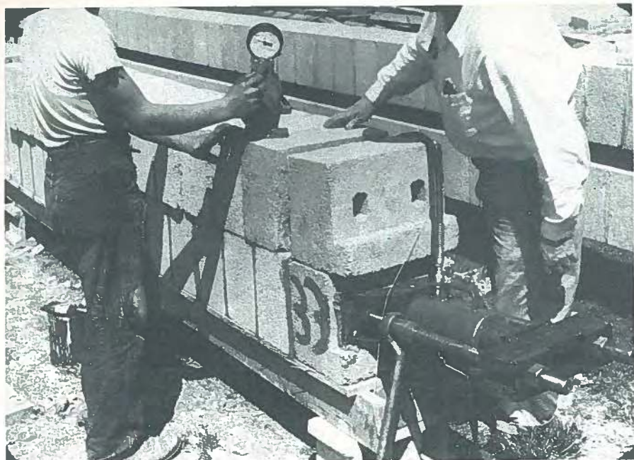
Fig. 2. Tensioning stadium beams.
