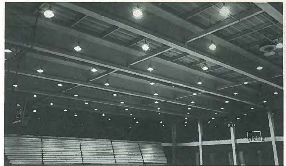
Fig. 42. Completed gymnasium with 120-ft clear span.
