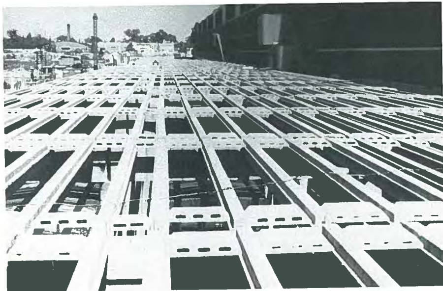
Fig. 13. Prestressed block joist and filler construction on 100,000 sq ft (9290 m 2 ) warehouse for Crosley Corporation. Joists are made continuous over 18 x 24-in. (457 x 610 mm) prestressed block beams by reinforcing steel in the topping slab.
