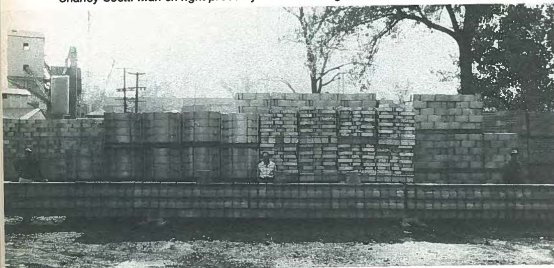
Fig. 17. Continuity test at Breeko Plant. On the left is Lloyd Markham, at center Charley Scott. Man on right probably carried loading blocks. Taken in August 1952.
