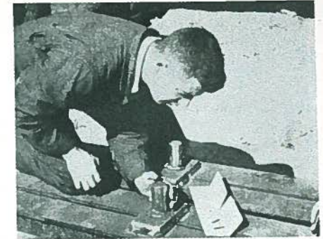
Fig. 4. The author examining the instrumentation during the testing of the Walnut Lane prototype girder.
