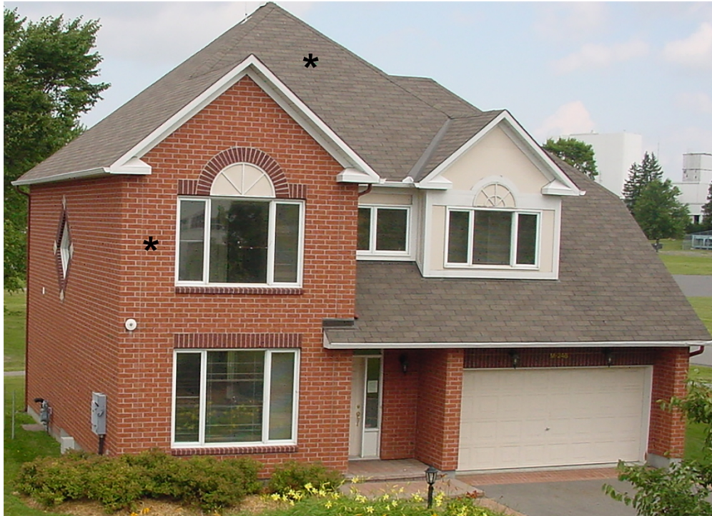
Figure 1. CCHT test house. Sensors location on wall and roof are indicated with a star.
