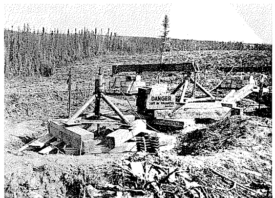
FIG. 6. Anchors under load at Thompson.
