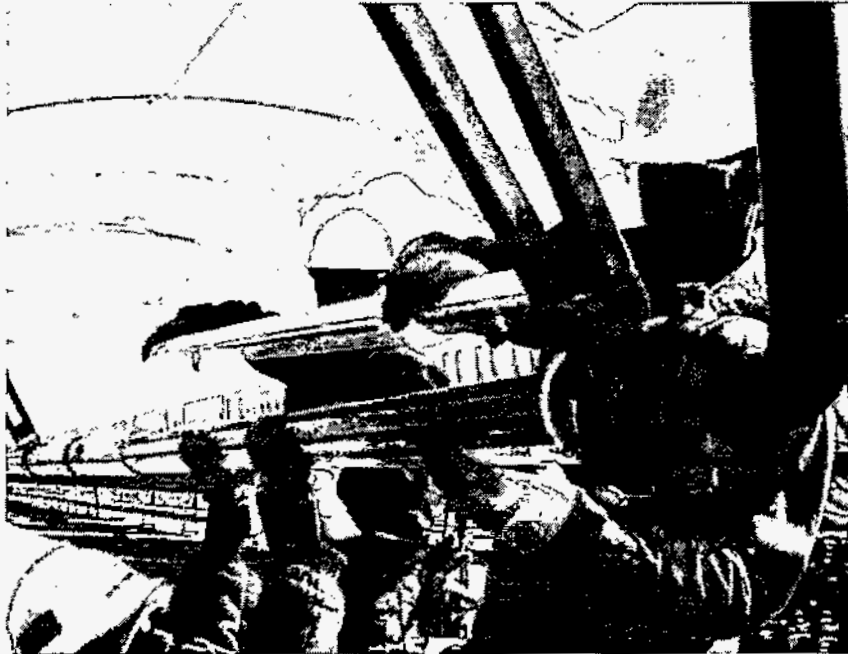
Figure 5. Split-glass envelopes were developed as a temporary method of reducing HCE heat losses.
