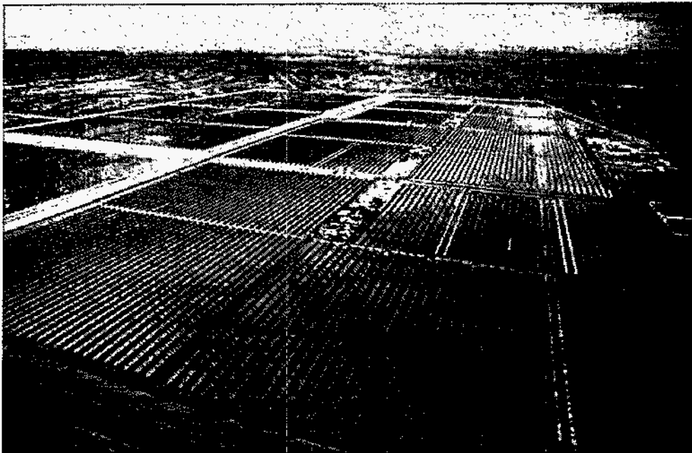
Figure 1. The Kramer Junction power park is comprised of five 30-MW plants.
