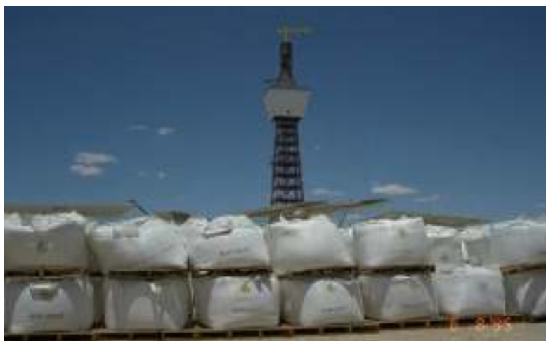
Figure L-2. 1000 kg bags of nitrate salt awaiting melting at Solar Two. The Solar One tower in the background is being prepared for installation of the new molten salt receiver.
