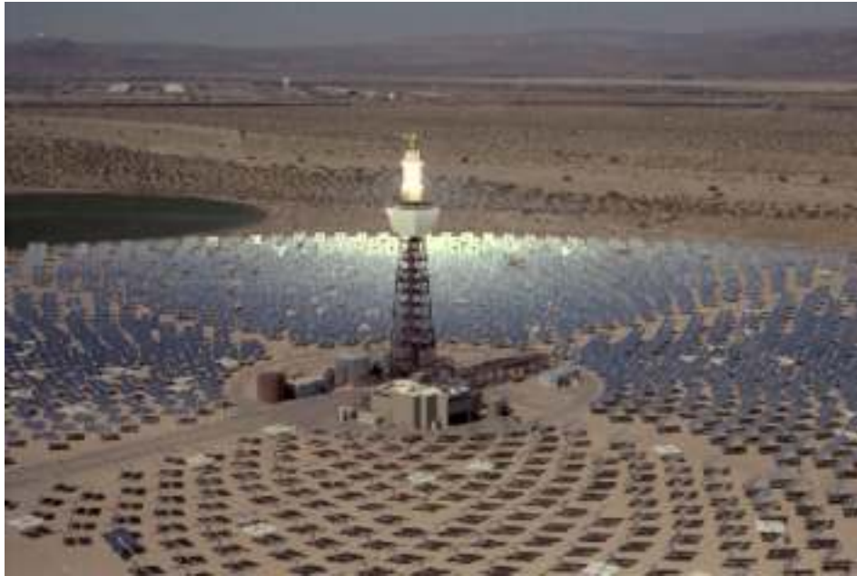
Figure 1-1. Photograph of the Solar Two plant in operation.
