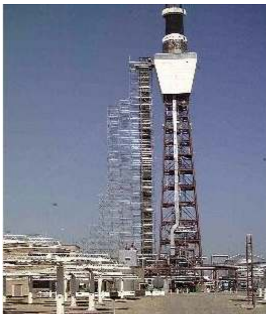
Figure 4-6. Chute on one side of the tower in which the nitrate salt was prilled for removal from the site.
