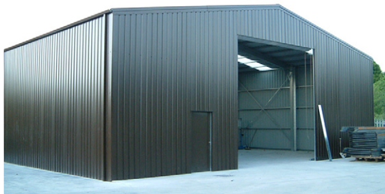
Figure 1. Typical cold-formed steel portal frame
