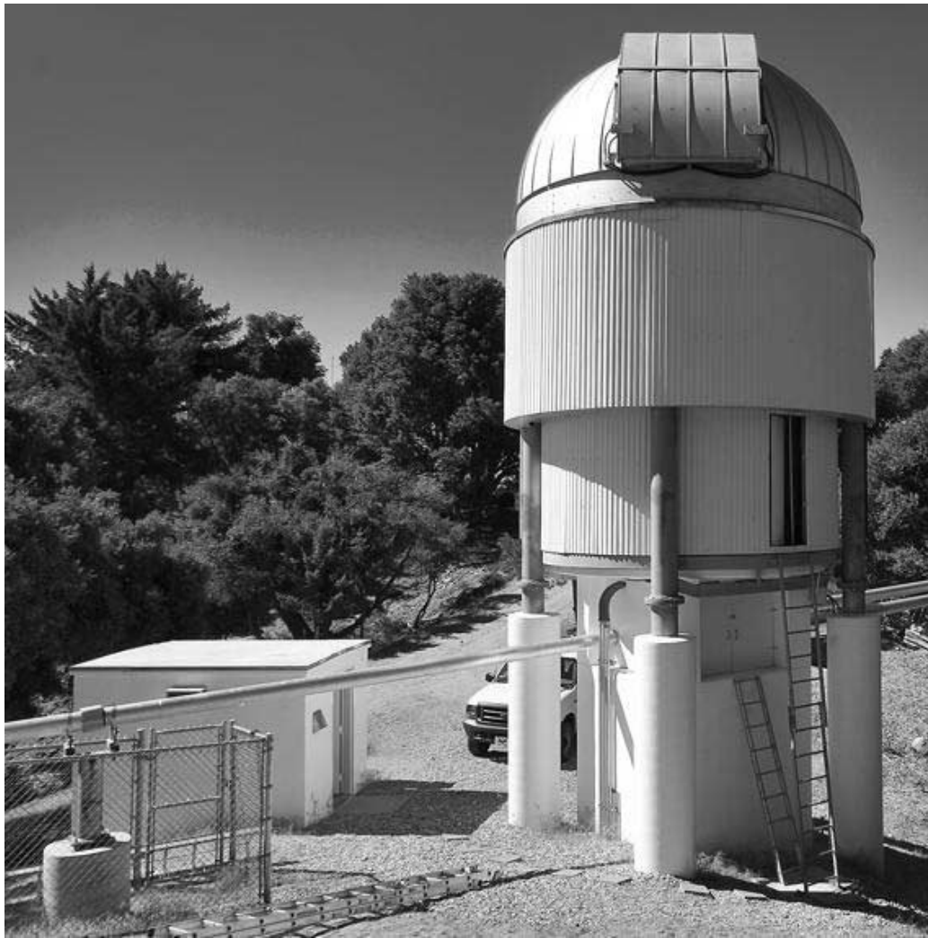
FIG. 5.—E2 telescope enclosure and electronics bunker. The small entry door can be seen on the right of the lower cylinder. Both the upper and lower cylinders can move to allow a free flow of air around the telescope. The light pipe from E1 comes from the left, passes through the coude area below the lower cylinder, and leaves to the right with the light pipe from E2. Photograph by Steve Golden.
