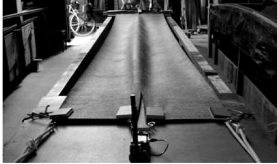
Figure 13 –Funicular shell formwork created by selective prestressing. Photo: Mark West (C.A.S.T.) [94].
