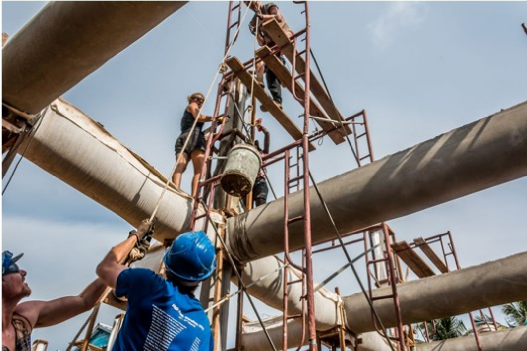
Figure 4 - Fabric formed beams and columns. Photo: Lindsay Perth.
