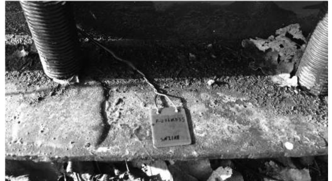
Fig. 12. Attached FSM transducer on the 4 m diameter tank floor without any surface preparation.
