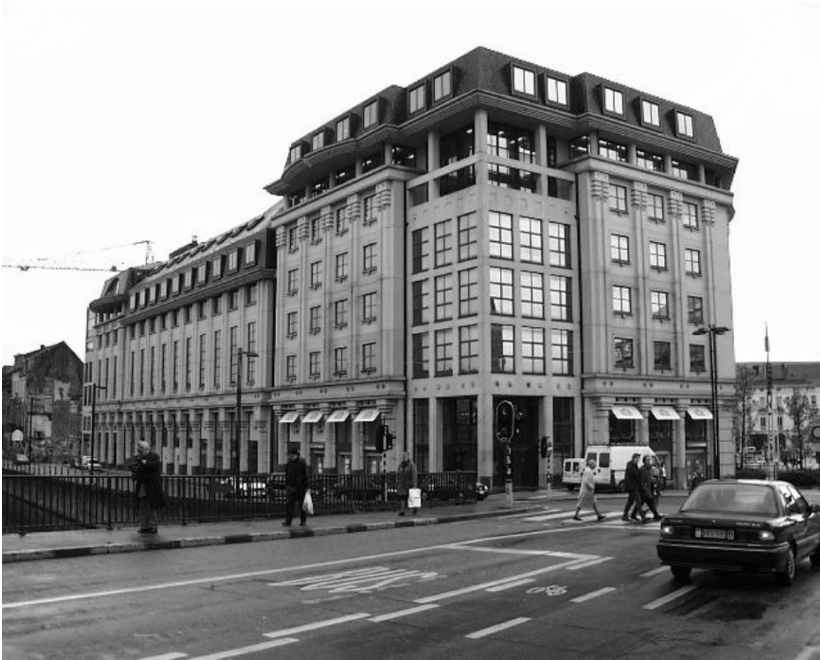
Fig. 7. The Urbis building in Ghent, Belgium.
