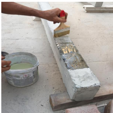
Fig. 4. Applying epoxy resin to concrete surface.
