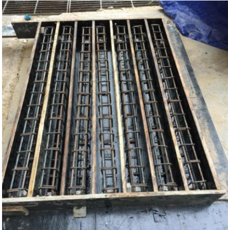
Fig. 3. Construction of RC beams.
