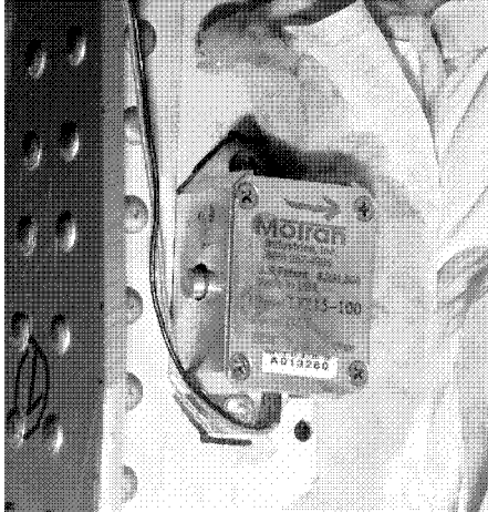
Figure 7. Inertial actuator mounted to 1900D frame.
