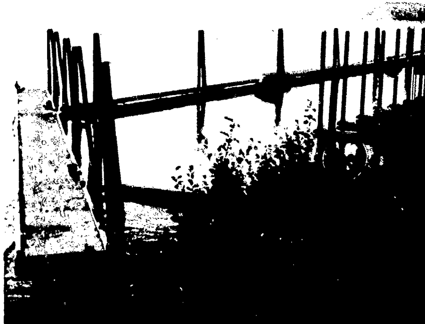
a. Floating breakwater section.
