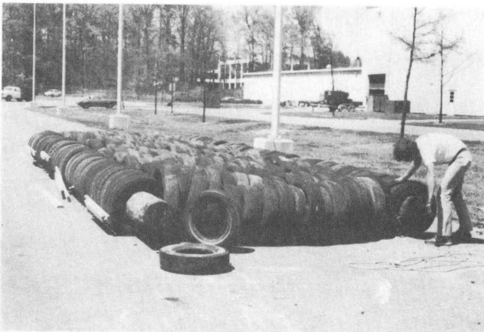
Plate 2. Assembly of PT-Breakwater. CBB790-14041
