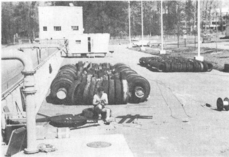
Plate 1. PT-Breakwater before testing at Coastal Engineering Research Center, Ft. Belvoir, Virginia: truck tires/steel pipe on left and automobile tires/telephone pole on right.
