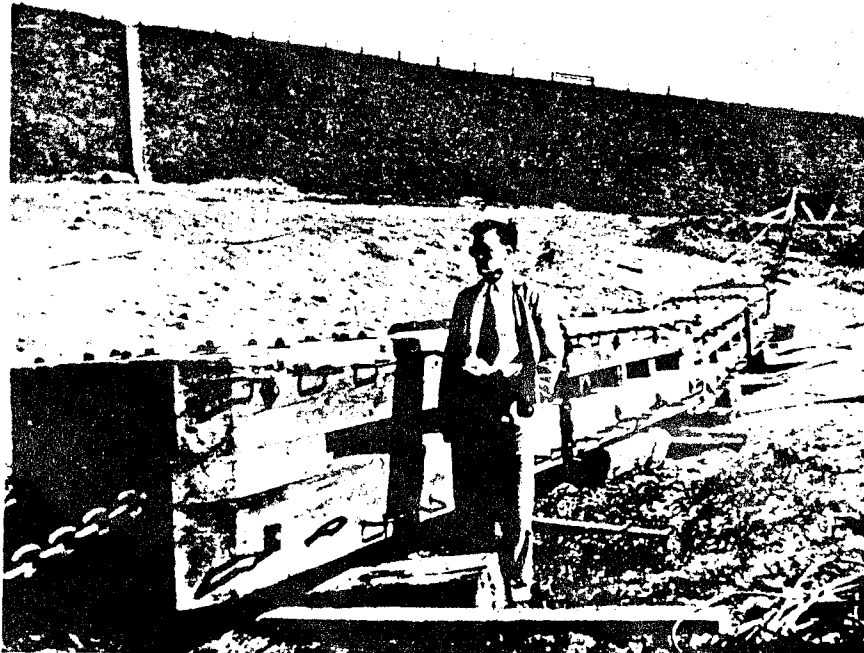
Fig. 12. Very Strong Deep Boom (Note the retainers for fence posts along the face.)
