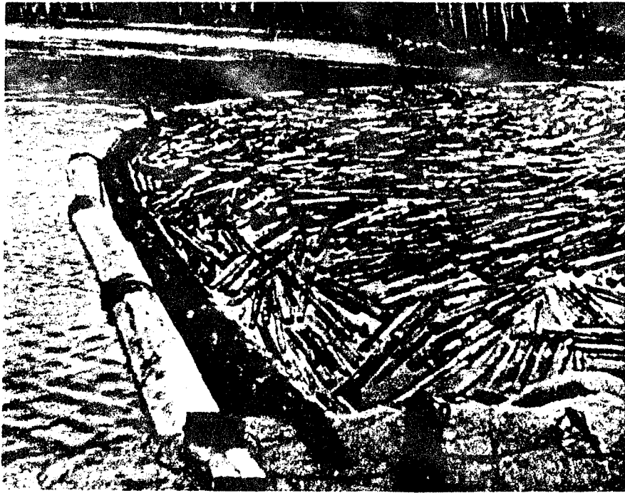
Fig. 7. Holding Boom Composed of Two Strings of Sitka Spruce
