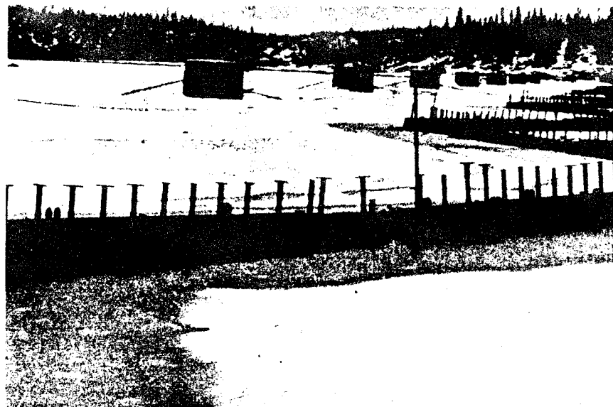
Fig. 14. Steel Pontoon Fence Boom in Winter Ice (Posts are lowered before wood arrives.)
