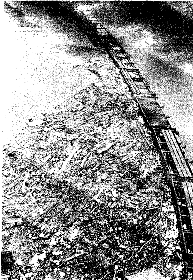
Figure 7. Debris diversion boom and debris, Appalachian Power Company Station at Winfield Lock and Dam, Kanawha River, West Virginia.
