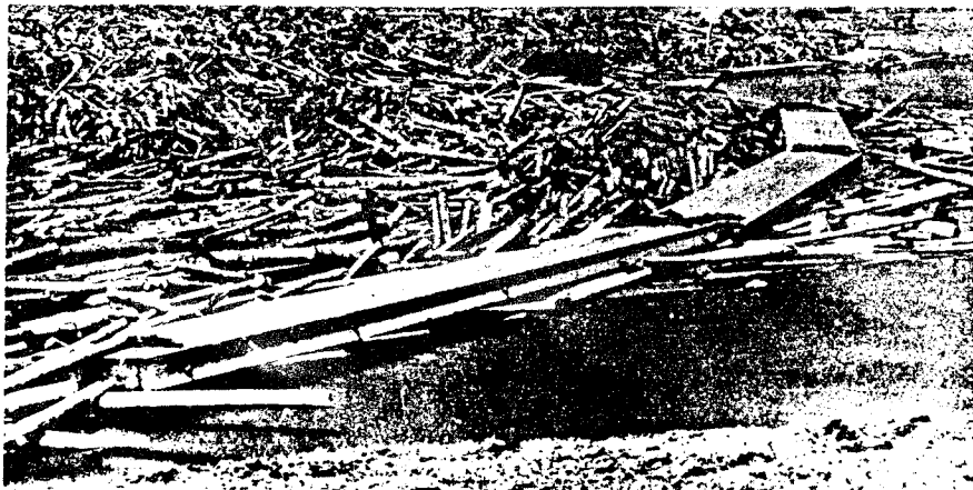
Fig. 10. Pulpwood Pushed Under a Flat Boom
