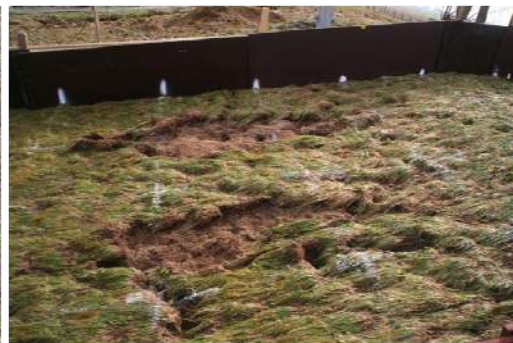
Figure 17. Various damaged locations
