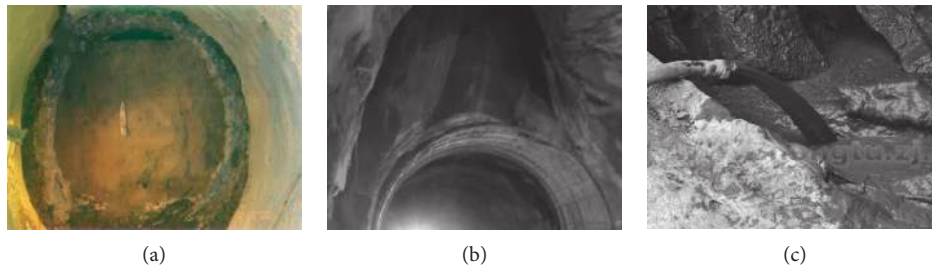
FIGURE 5: (a) Bolu highway twin tunnel [240], (b) collapse, and (c) treatment with pumped FC in Shima tunnel [241].
