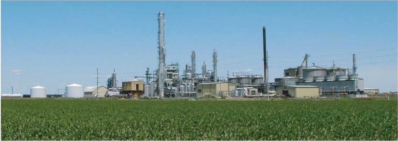
Figure 1. A maize grain-ethanol biorefinery in Hastings, Nebraska, which uses about 0.6 million tons of grain annually to produce 250 million liters of ethanol.
