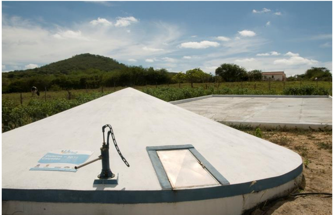
Fig 1. Boardwalk Cistern, a 52,000 liters water tank connected to a boardwalk that captures rainwater [16].
