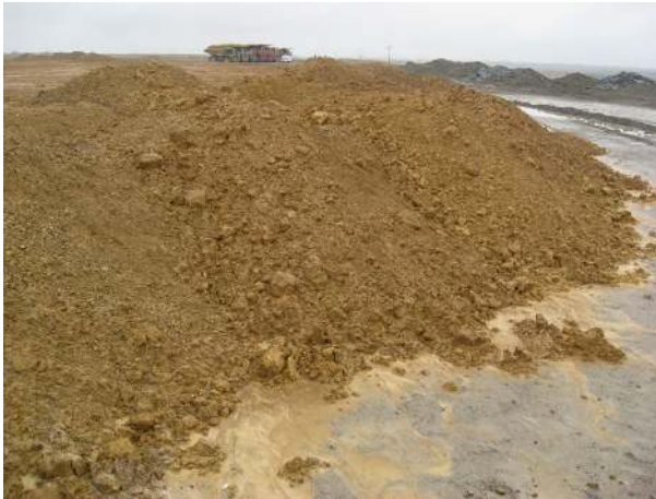
Fig. 2 Soil replacement following coal mining on a reclamation site in southwestern Indiana, USA. Operational procedures in this region call for level grading of the replacement soil followed by planting of native hardwood trees. Photo credit: D.F. Jacobs
