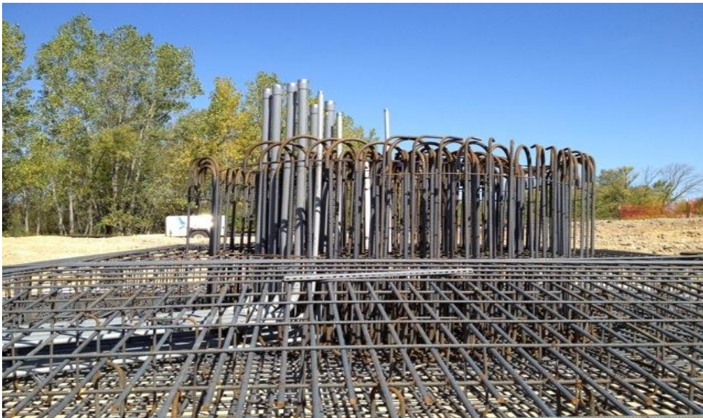
FIG. 2.1 Reinforcement in shallow octagonal foundation (Courtesy of Stephen Schubert).
