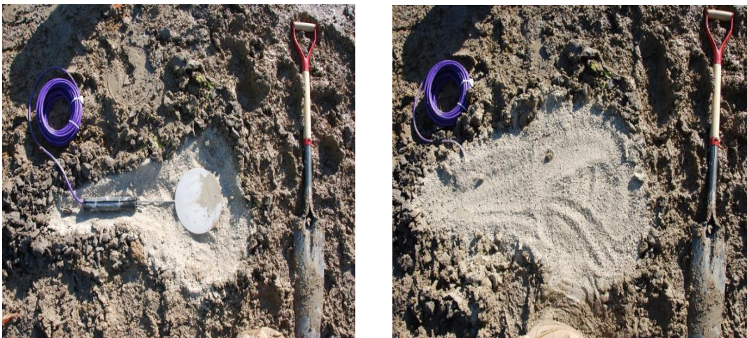
FIG. 3.13 Pressure cell installation.
