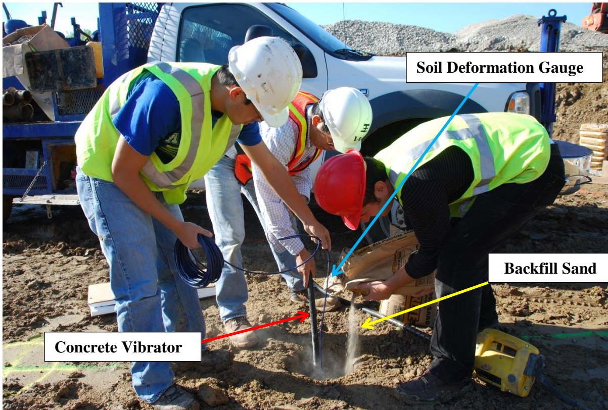
FIG. 3.17 Soil deformation gauge installation.
