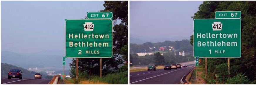
Fig. 7.3 The previous standard font, Highway Gothic ( left ) and in the ClearviewHwy font ( right ). These signs are on I-78, near Allentown, PA. The Clearview has larger holes in letters like e and o, and slightly more readable serifs on letters like l and t. The text is particularly more readable at night when illuminated by headlights. (Photos © Don Meeker and used with permission)
