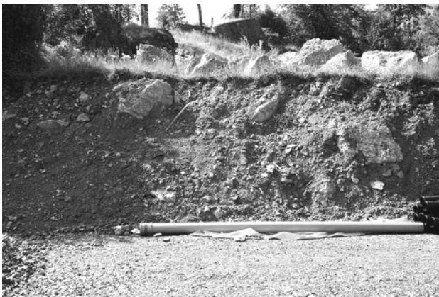
Fig. 3 Present day view on a road-cut through the upper few metres of the deposit of the Goldau sturzstrom of 1806, close to the zoological garden in Goldau (514 m a.s.l.). The quasi-matrix supported fabric of the highly fragmented conglomerate is clearly visible. Note the accumulation of large blocks on top (the 5 m long tube in front serves as scale)
